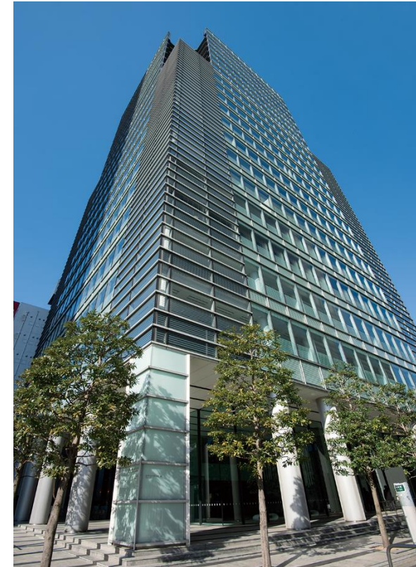
Head Office : 1-30-5 Hamamatsucho, Minato-ku, Tokyo Hamamatsucho Square
